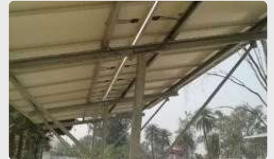
130kWp Solar Car Park Shed at Teva, Gajraula, Uttar Pradesh.
