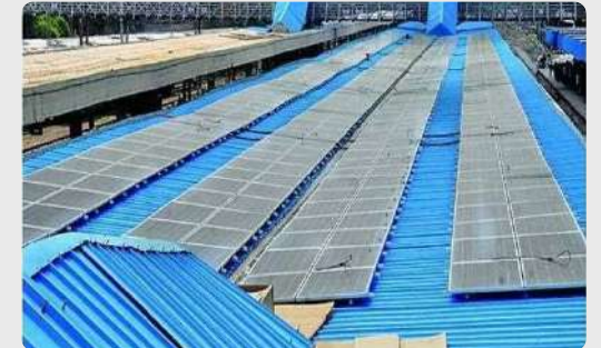
1.5MWp Solar Project at Kanpur & Allahabad Railway Station.
