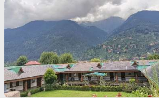
2.5MWp Solar Project for Club Mahindra Group, Pan India.
