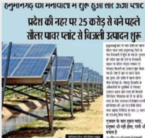
Asun Solar set up the first canal-top project in Rajasthan with a 2MWp capacity.
