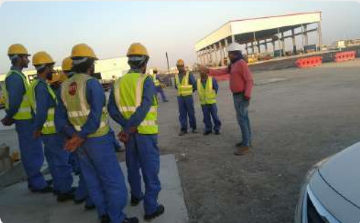
1.3MWp Solar Project for OMASCO, Oman.
