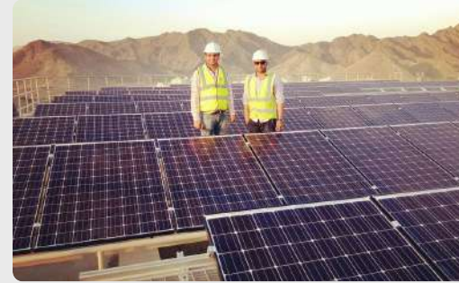
55kWp Solar Project for Mazoon Electricity, Muscat (Oman).
