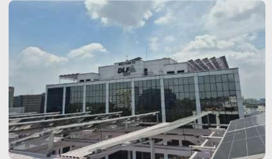
185kWp Solar Project at DLF Corporate Park, Gurgaon.
